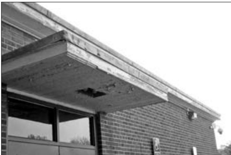
Fascia board will be replaced at Parkville .
